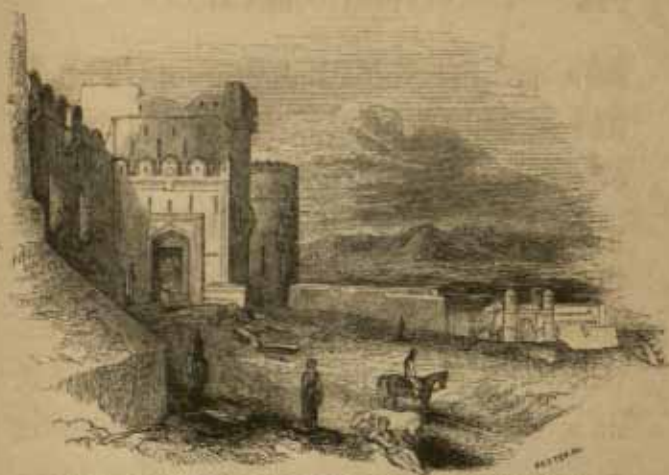
GATE LEADING INTO THE FORT AND TOWN OF AITOK, LOOKING WEST.
