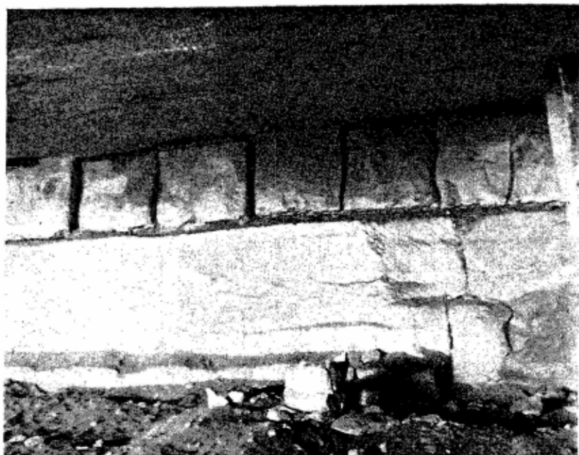
1(c) Ancient Egyptian quarry showing method of quarrying stone
