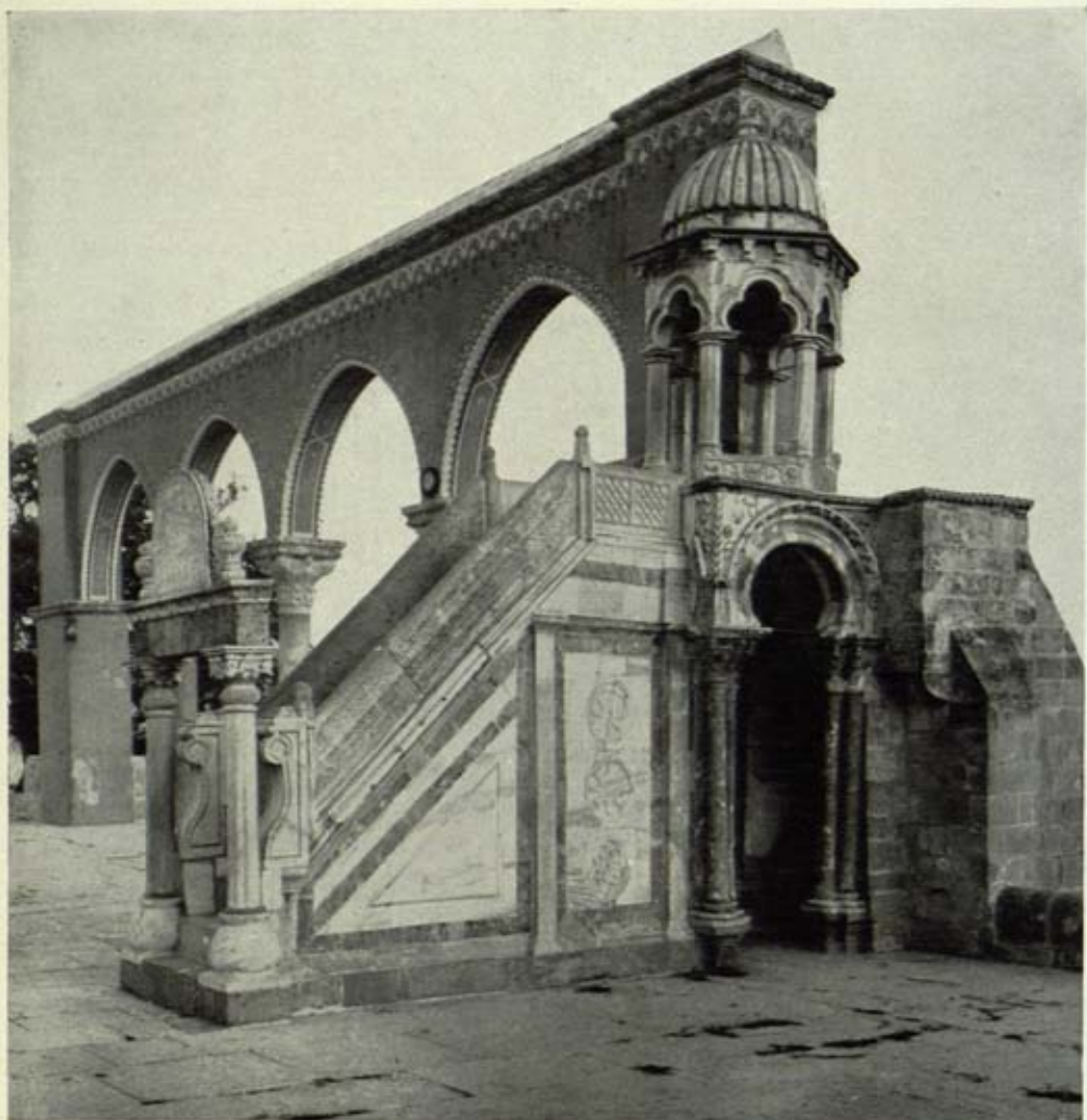
[98] Pulpit of Judge Burhan-ed-Din, dating from 1525. It was formerly used for prayer on high feast days and for rogations for rain. This graceful open-air minbar contains numerous fragments from former monuments, both Byzantine (capitals flanking the staircase gate) and Frankish (small columns supporting the pulpit itself).
