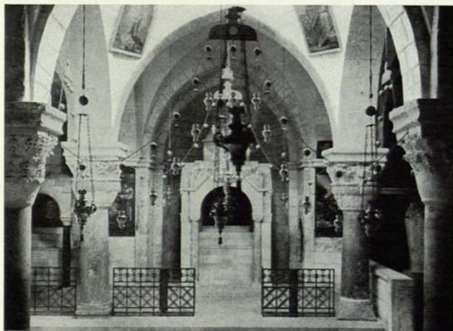
[76] INTERIOR OF THE CHAPEL OF SAINT HELENA. Situated below the Holy Sepulchre, and similar to a crypt, its architectural styles are oddly composite: parts of ancient columns narrower than their capitals of Byzantine origin (two of which are 'vase-shaped'); vaulting probably reconstructed during the Crusades. During the Middle Ages innumerable pilgrims left records of their visits to this chapel in the form of little crosses carved into the entrance walls.
