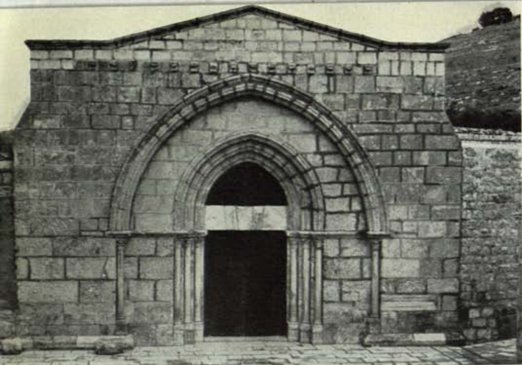
[127] FAÇADE OF THE TOMB OF THE VIRGIN. The ancient crypt is the only remaining part of the Abbey of Our-Lady-of-Jehoshaphat, founded by Godfrey of Bouillon, and destroyed by Saladin. Its portal is without doubt the most typically Western monument in Jerusalem, with a double pointed or broken archway.
