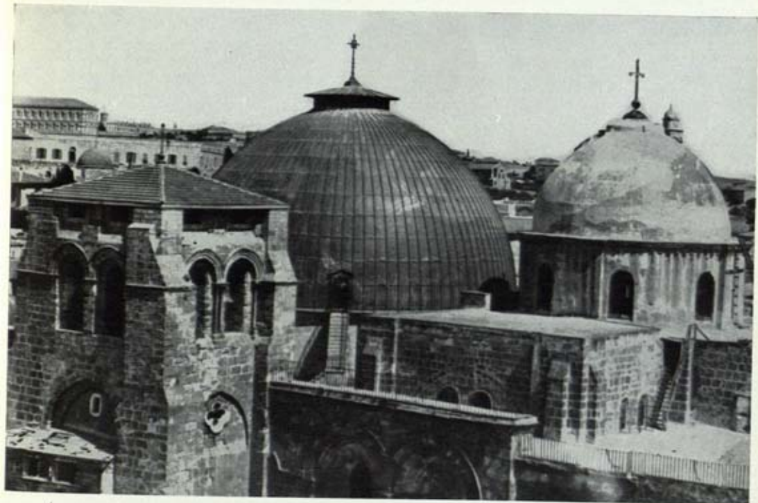
[106] The bell-tower and two domes of the Holy Sepulchre. The twelfth-century tower is today incomplete. The large dome has an ugly covering of zinc painted black and dates from the restorations of 1809. It is above the former, transformed, Anastasis. The rest of the building, on the right, consists of the transept with the principal façade, the dome dating from the Crusades, and the choir, and was the work of the Franks, finished in 1149.
