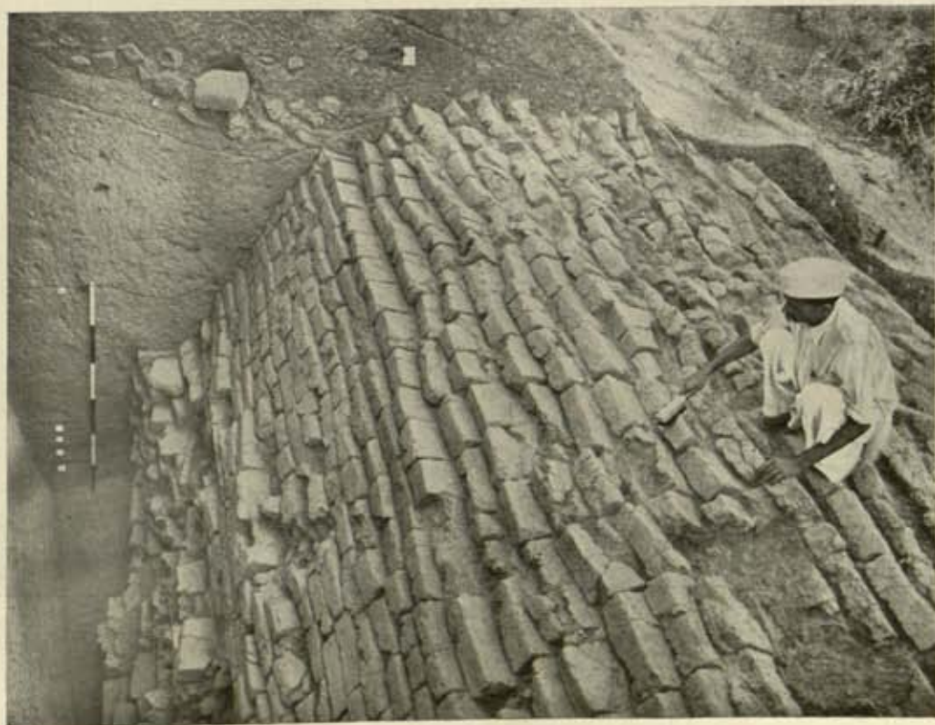
B. Cutting SP II: fallen (outer) brick-revetment of Phase III
