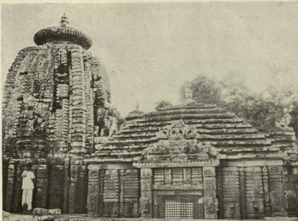
A. Muktesvara temple, Bhuvanesvar, District Puri, Orissa: lichen covering almost the whole of the vimāna and parts of the jagmohan in sporadic patches
