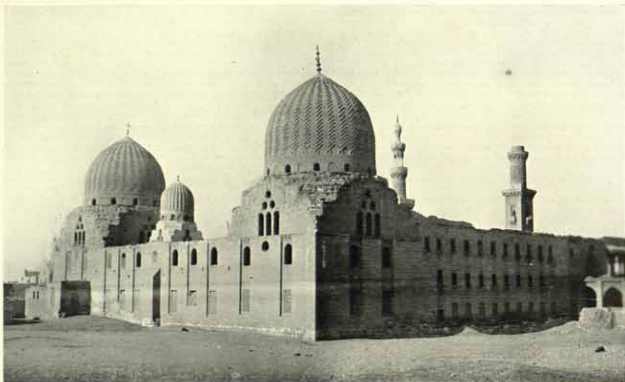
FIG. 97. EXTERIOR FROM THE EAST
