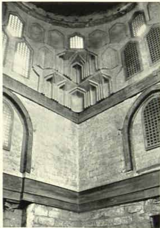
FIG. 75. CAIRO Mausoleum of An-Nāṣir intra-muros . Dome
