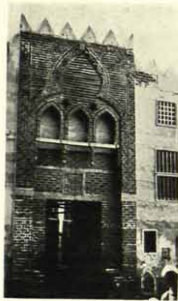
FIG. 145. ROSETTA Mosque of Alt 'Al-Mahalli Doorway
