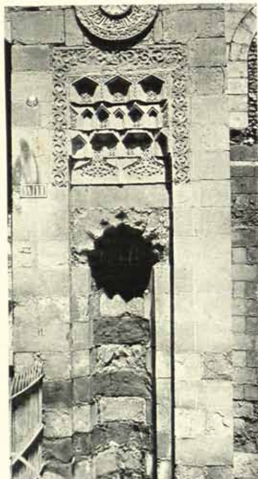
FIG. 59. CAIRO: MOSQUE OF BAYBARS I. Detail of south-west porch
