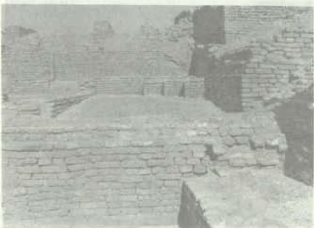
Fig.4 VS-A, Southern Part, showing modern retaining walls
