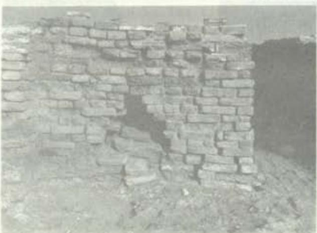
Fig.5 MN area, showing holes in the walls for the installation of horizontal isolation
