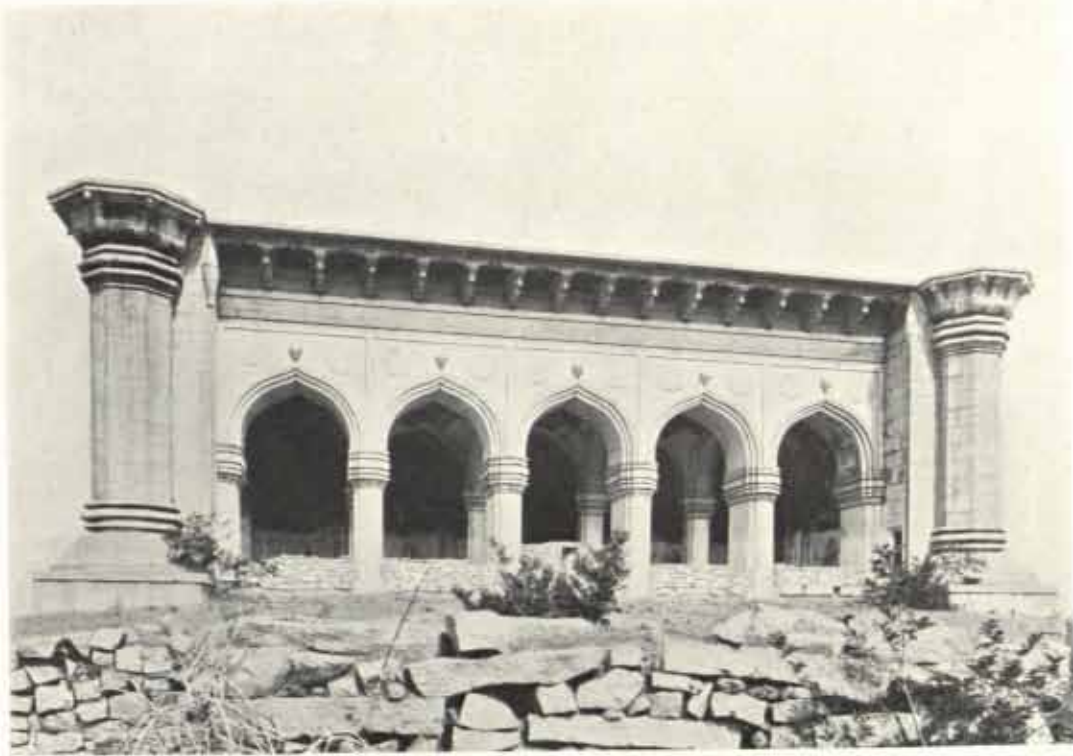
(a) MOSQUE OF PEMA MATI NEAR GOLCONDA: FACADE
