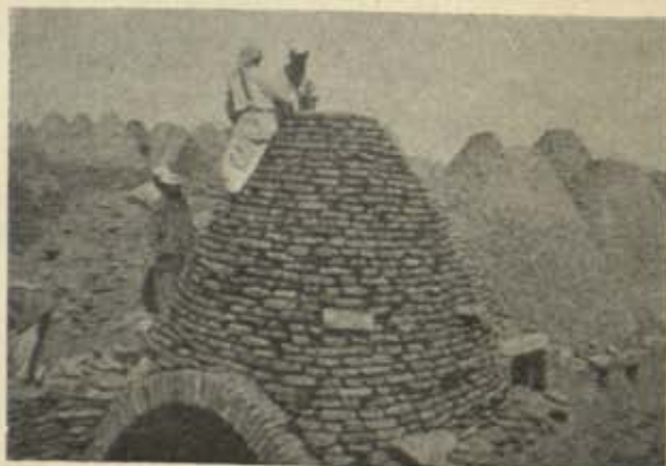
FIG. 5. MASON COMPLETING THE CORBELLED DOME Note the corbelled pendentive, built to accommodate the next dome.
