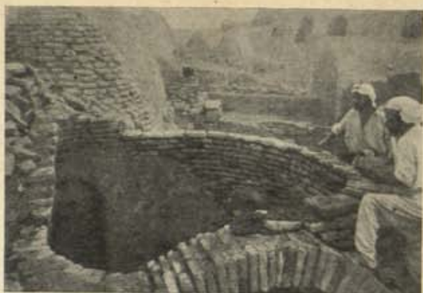
FIG. 3. JUNCTION OF DOME AND TRANSVERSE INTERNAL ARCH
