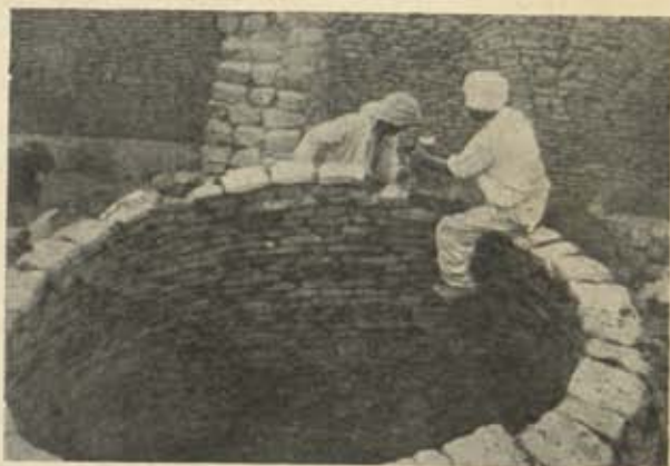
FIG. 4. INTERIOR OF A CORBELLED DOME IN COURSE OF BUILDING
