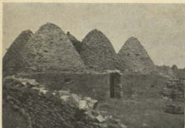
FIG. 2. HOUSE ROOFED WITH CORBELLED DOMES Haran, September, 1947: photographs by W. C. Brice
