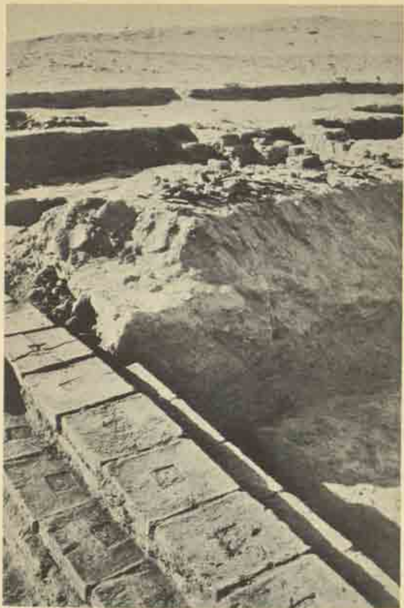
SO PROUD OF HIS DRAINAGE SYSTEM WAS AN EARLY SOVEREIGN THAT HE BUILT IT WITH STAMPED BRICKS
