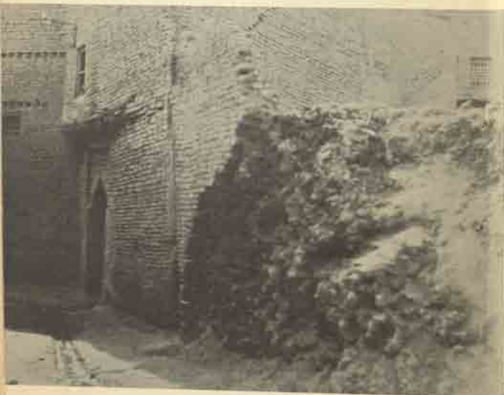
A CRUMBLING MUD-BRICK WALL IN A MODERN NEAR EASTERN CITY
