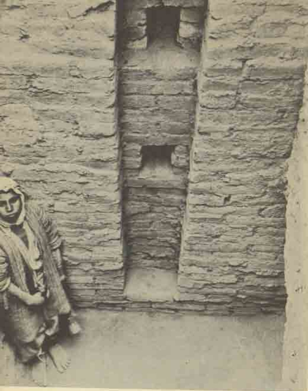
ANCIENT WALL CONSTRUCTION AND DRAINAGE CHANNELS
