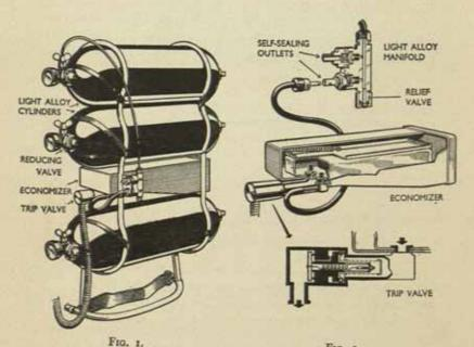
THE OPEN-CIRCUIT APPARATUS.
