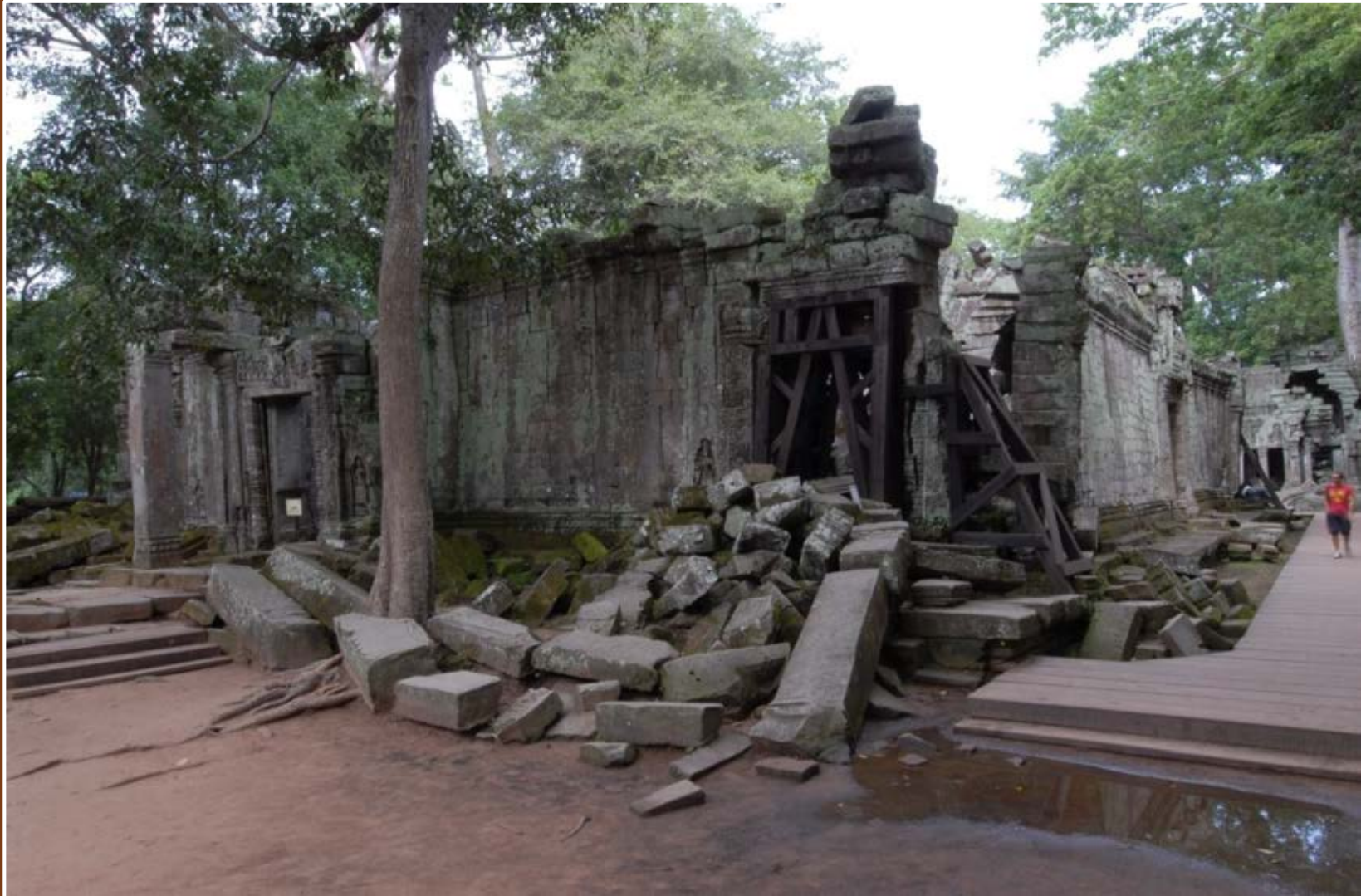
North-east corner before dismantling inclined wall and removing fallen stones
