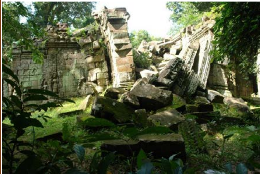
South Gate - facing North
