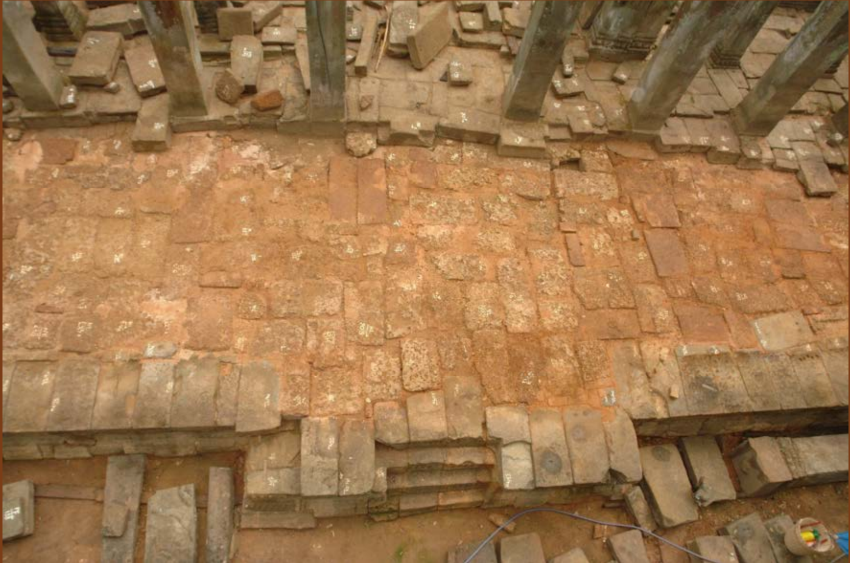
Hall of Dancers - Re-laying of interior northern laterite core after consolidation.
