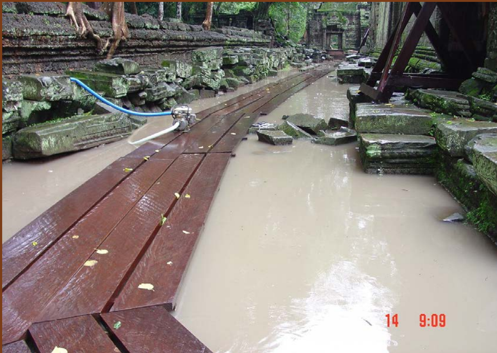
Stagnated Water in TA-PROHM, TEMPLE Archaeological Survey of India
