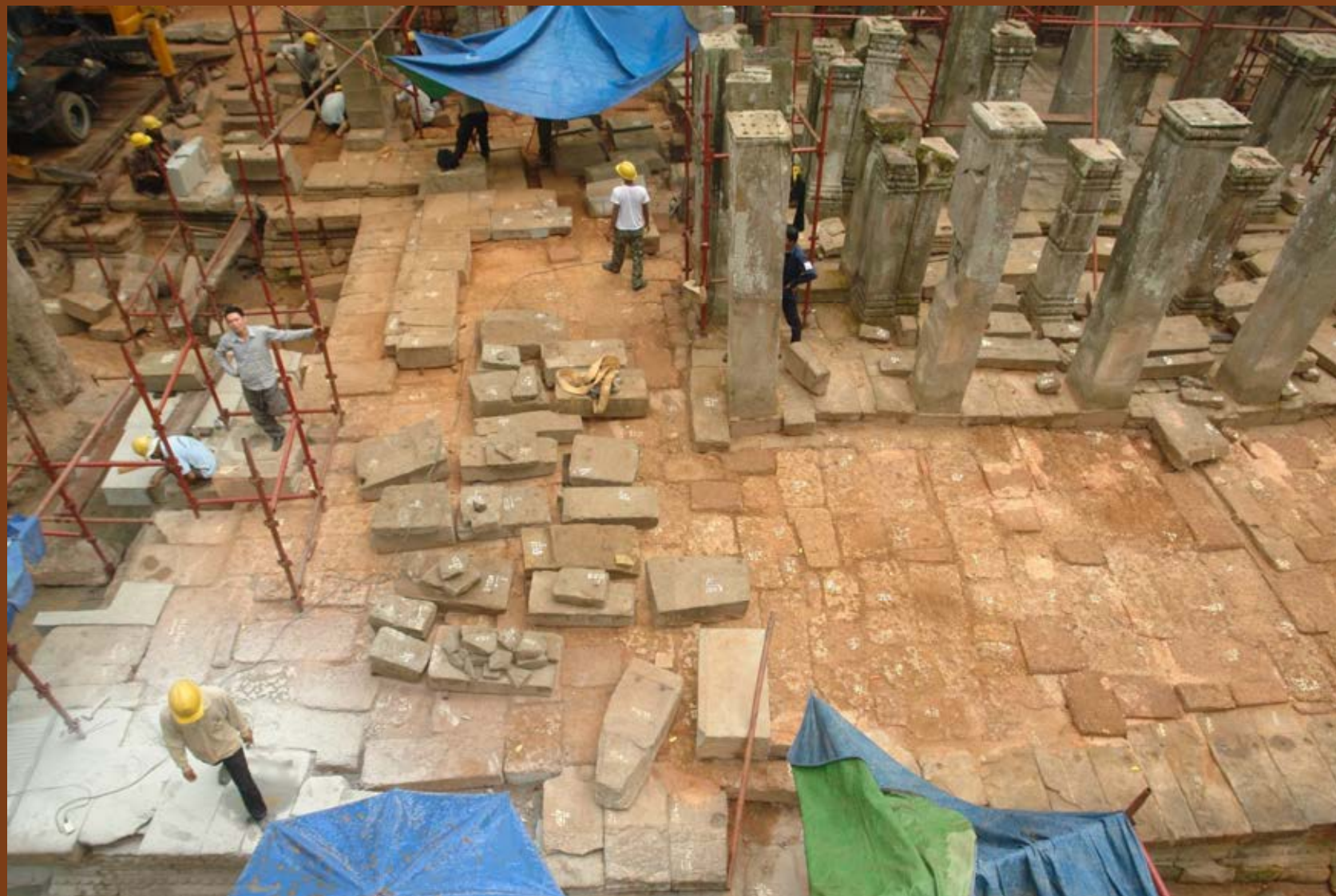
Hall of Dancers - Resetting of sand stone wall on eastern side.
