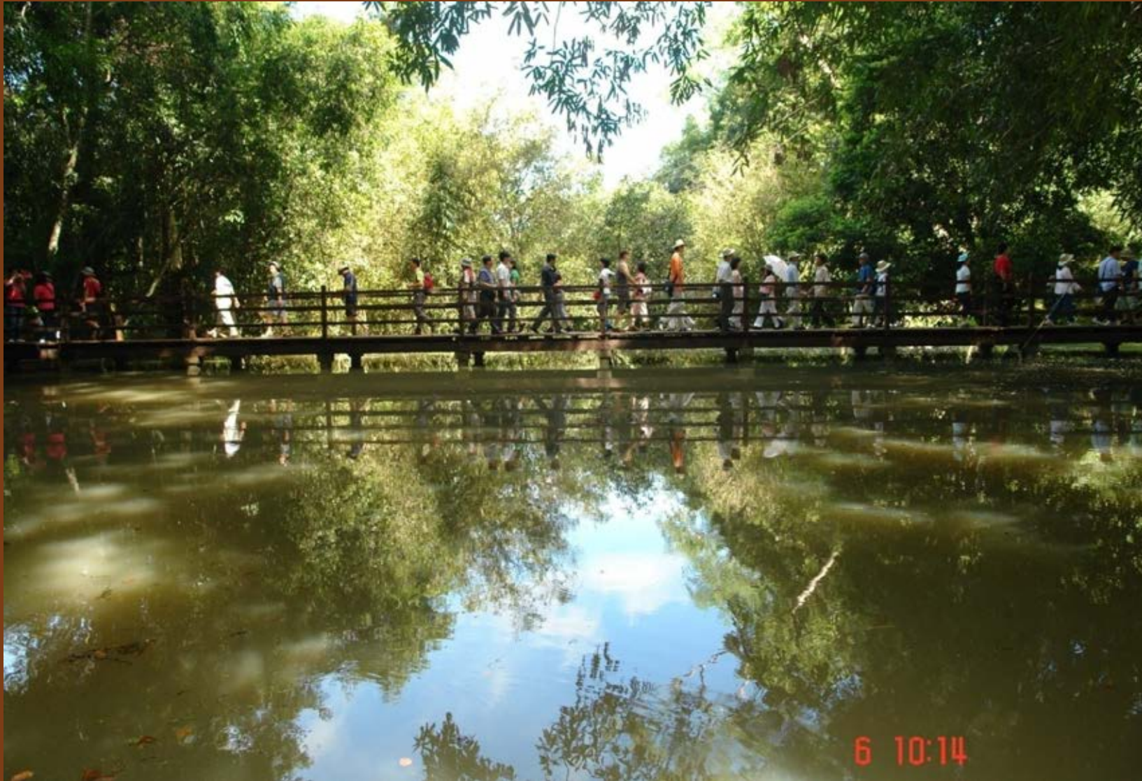
Wooden Bye-pass Bridge over Outer Moat (West side), Ta- Prohm , Temple Archaeological Survey of India
