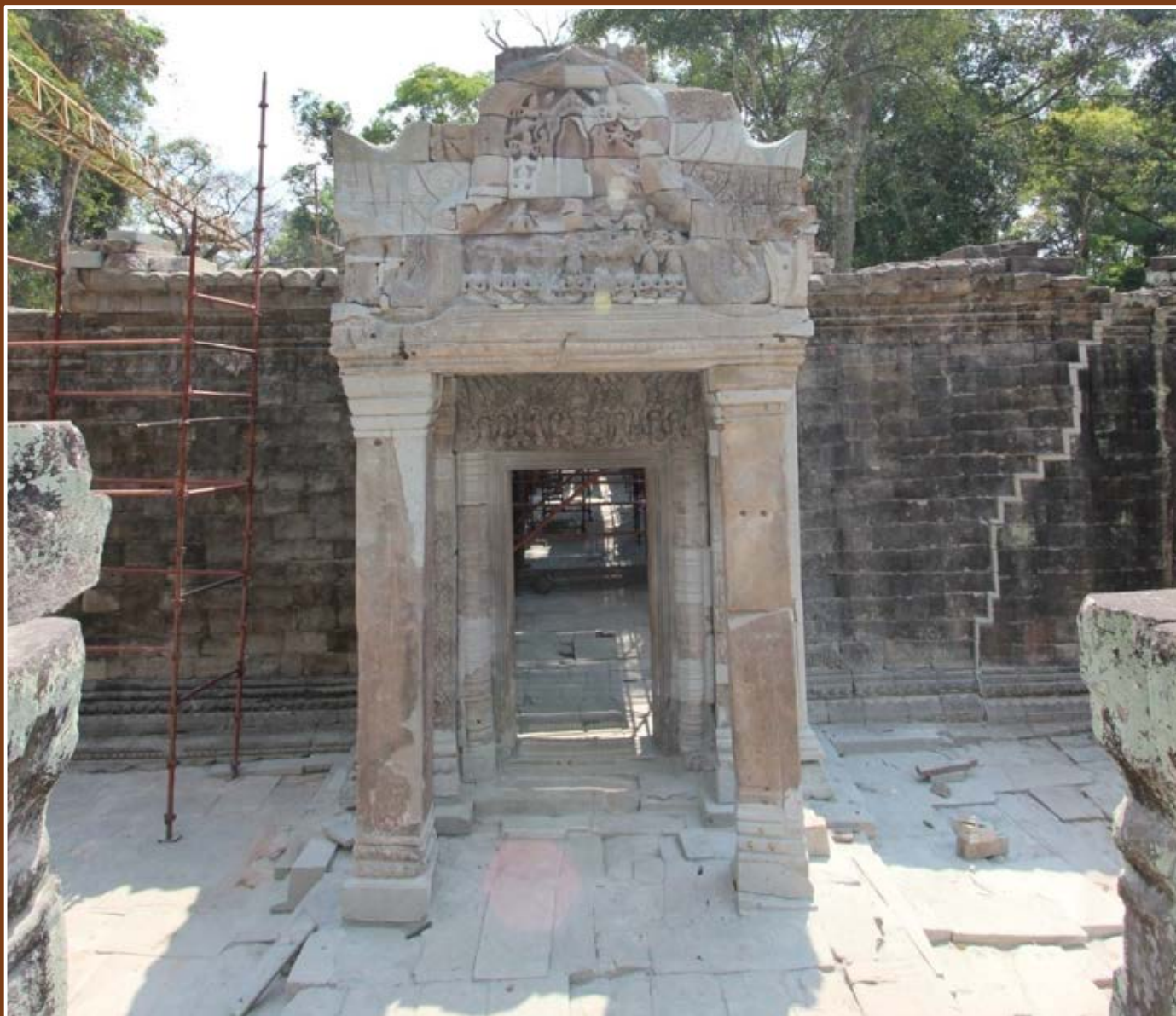
South-west Corner (Discernible distinction - original and restored portions)
