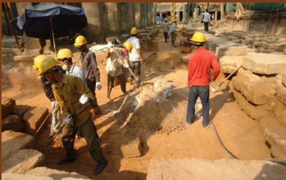
Hall of Dancers - Consolidation of interior northern floor foundation.
