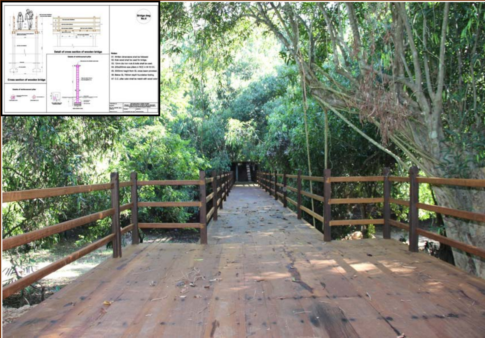
Construction of bye pass bridge for exit from south
